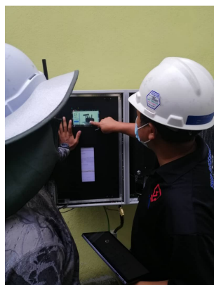
Installation of online gas monitor at TNB substation
