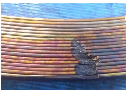
Short circuit of winding conductor
