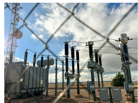
Installation of lightning arrester at transformer bushing
