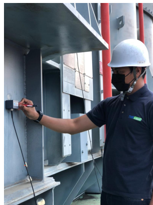
Installation of acoustic sensor
