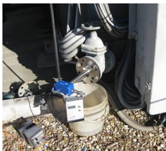
UHF probe install in oil drain
