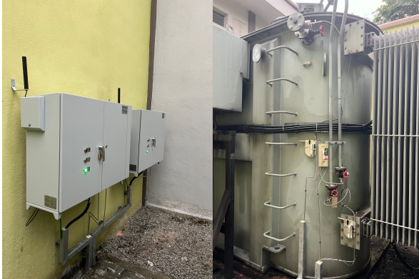
Installation of DGA online monitoring system at TNB substation
