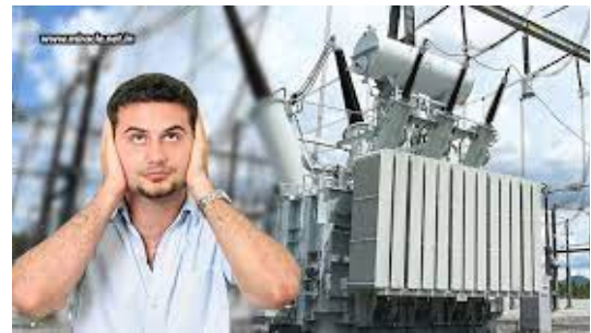
Noise generated by transformer
