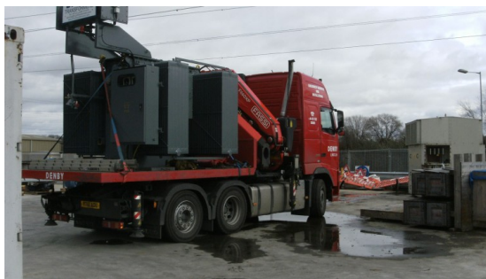
Transportation of fully assembled power transformer
