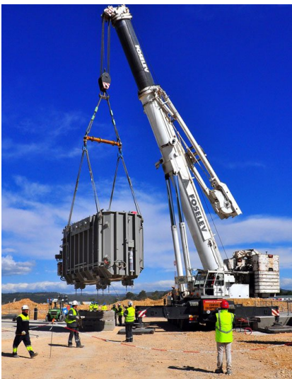
Transformer installation at site
